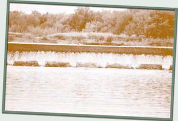
way to deal with erosion is by placing grade control structures throughout the wash, which are designed to lessen bank cutting by stormwater flows. After an in-depth study, several types of grade control structures have been identified for bank and channel stabilization efforts in the Wash. In total, 22 structures will be required to stabilize the Wash. Two structures were recently completed, and another is currently under construction.
