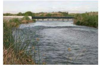
Weirs and vegetation help slow flows allowing sediment to drop out of the water column
