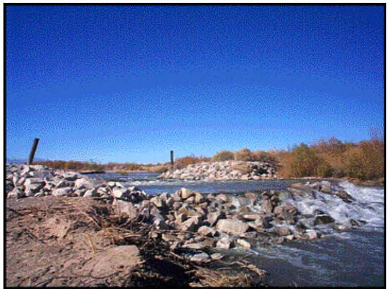
**Figure 1.7 - Photo of the Grade Control Structure after October 1998 emergency repairs were conducted (Southern Nevada Water Authority).**
