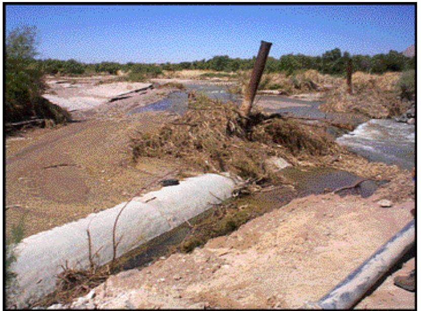
**Figure 1.6 - Photo of the Grade Control Structure after the September 1998 flood event (Southern Nevada Water Authority).**
