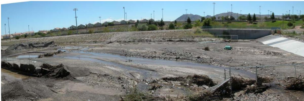
**Figure 2: Storm damage caused by the August 14, 2005, flood event. The image was taken from the same overlook as Figure 1. Sediment, storm debris and surface flows cover what should be the SSF cell in the foreground.**
