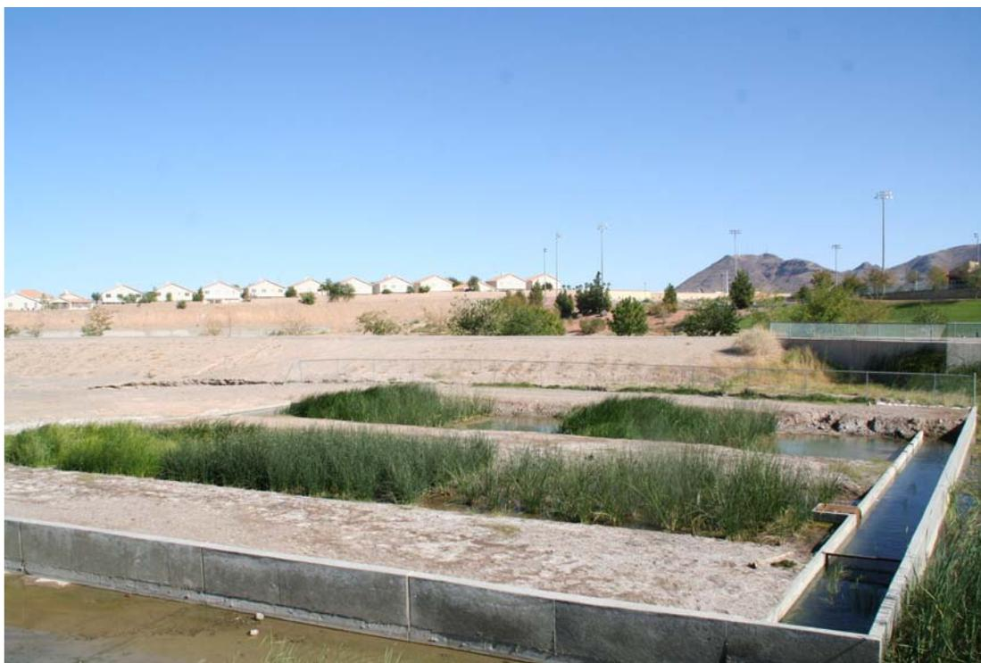
**Figure 3: October 12, 2006 site overview looking southeast with the SSF cell in the foreground. Note the standing water visible in the SSF cell.**
