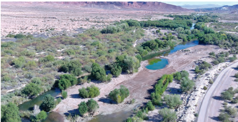
BOR grant project area downstream of Pabco Weir after sediment removal
