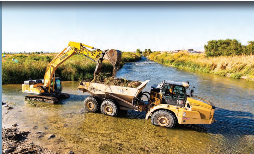
Crew conducts maintenance clearing in the impoundment of Upper Diversion Weir
