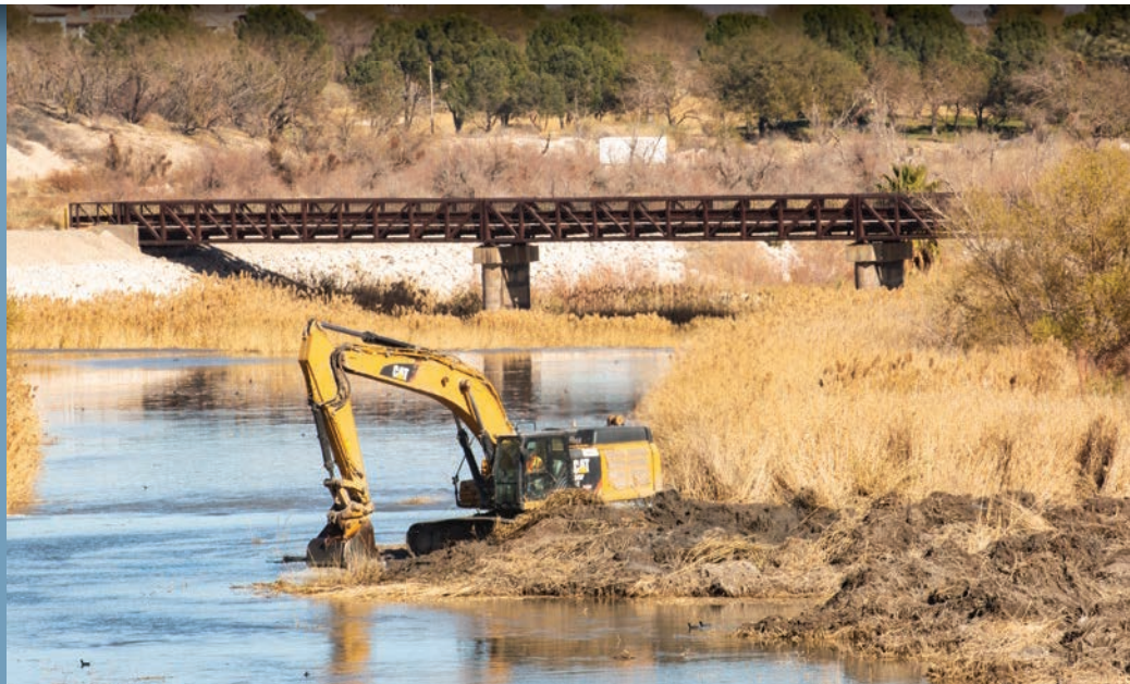
Vegetation removal above Powerline Crossing Weir
