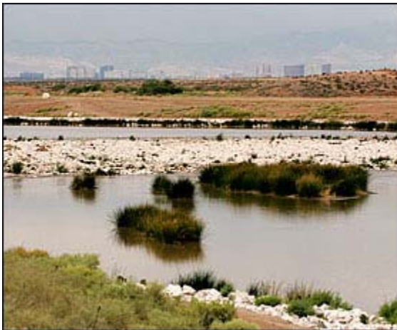
The Lower Narrows Weir from the Wells Trailhead.
