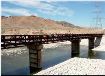
Powerline Crossing Bridge
