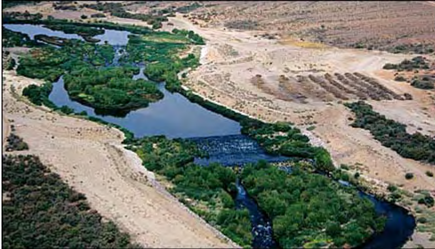
Aerial view of two weirs and associated revegetation
