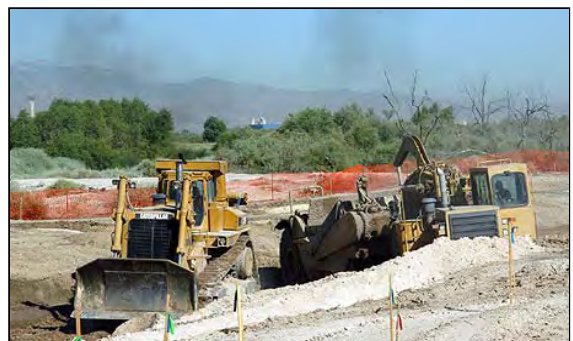
Construction equipment removes soil near the future Upper Diversion Weir site.
