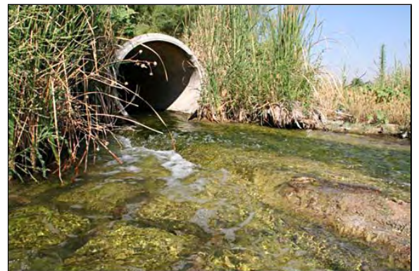
Water quality samples were taken every half-mile and at each dewatering source testing for selenium.
