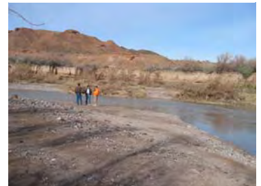
Site of the future Powerline Weir
