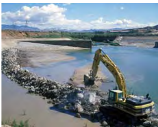
BOR crews installing bank protection at the Rainbow Gardens Weir in 2005
