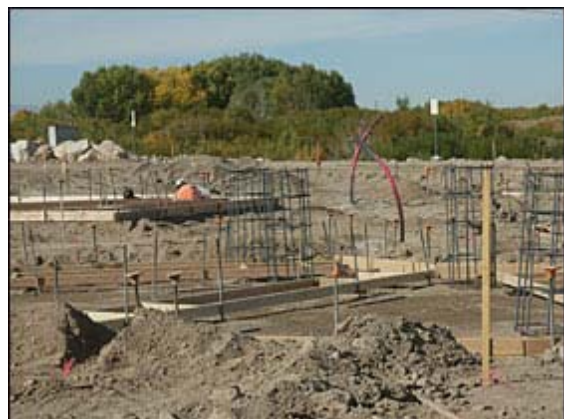
Construction has begun on the future Pabco Road trailhead.
