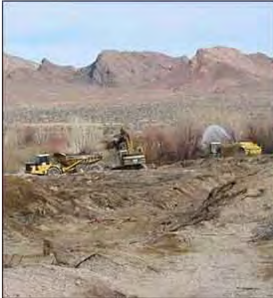
Reclamation construction crews clearing vegetation in 2008.
