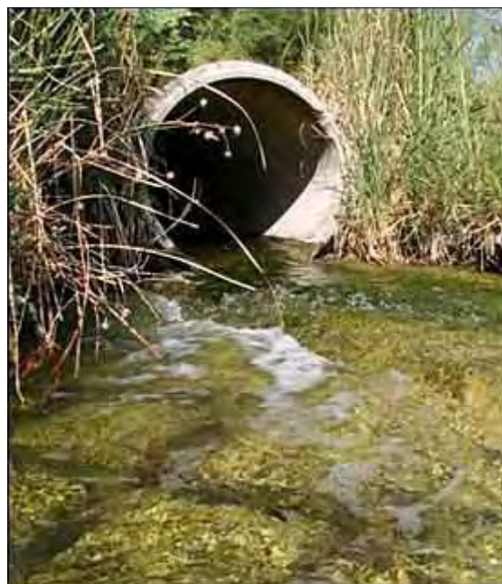
A dewatering pipe in one of the area tributaries.
