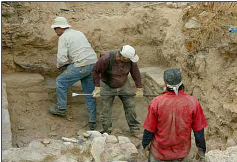
Stone slabs are mapped, marked, carefully removed and prepared for relocation to the Clark County Museum.
