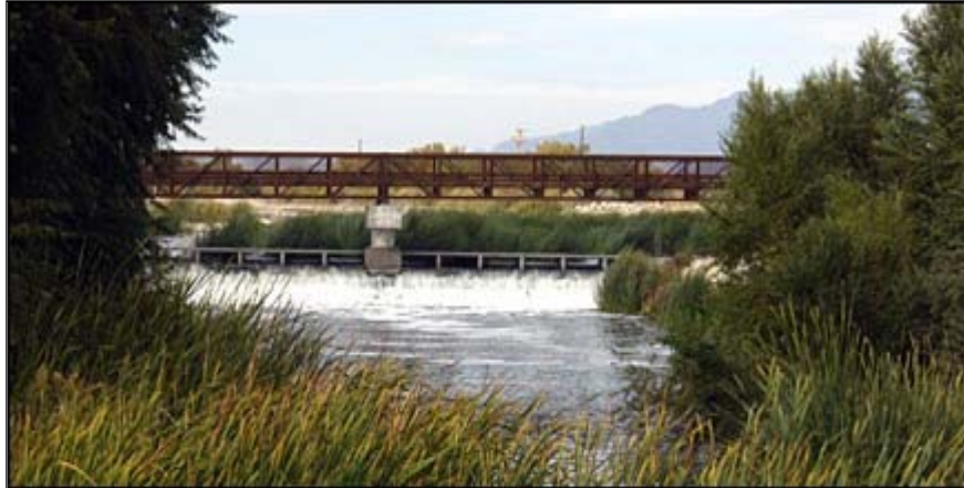
The Upper Diversion Weir and bridge was recently awarded the APWA Environmental Project of the year.
